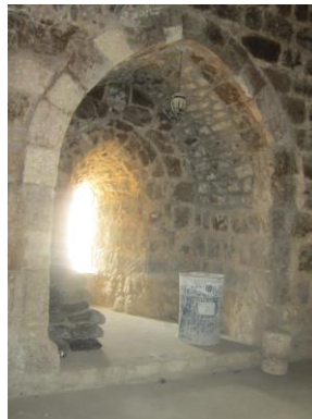
Figure 22. Groin vault, can be thought of as the intersection of two barrel vaults
