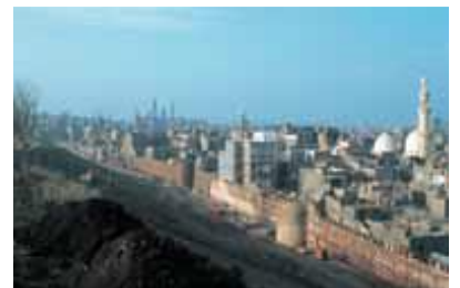
Figure (9) Ayyubid wall Restoration
