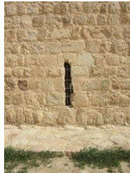
Figure 21. As defensible space small openings, (arrows)
