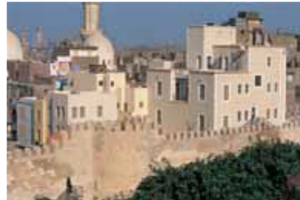
Figure 12. Housing rehabilitation in Darab Alahmar Neighborhood
